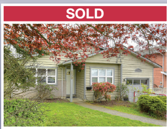
659HessCrescent.com SW Glandford
